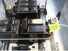
Step 7: Re-Install panel cover, Verify proper operation of interlock. Main breaker **ON**, generator breaker **OFF** and generator breaker **CAN NOT** be turned on. Generator breaker **ON**, main breaker **OFF** and main breaker **CAN NOT** be turned on. Please verify that inside panel cover is touching all breaker, if not adjust panel cover with top and bottom screw on cover.
