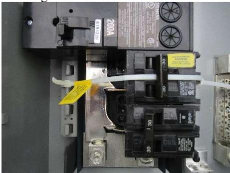
Step 7: Re-Install panel cover, Verify proper operation of interlock. Main breaker **ON**, generator breaker **OFF** and generator breaker **CAN NOT** be turned on. Generator breaker **ON**, main breaker **OFF** and main breaker **CAN NOT** be turned on.
