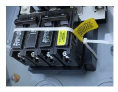
Step 7: Re-Install panel cover, Verify proper operation of interlock. Main breaker **ON**, generator breaker **OFF** and generator breaker **CAN NOT** be turned on. Generator breaker **ON**, main breaker **OFF** and main breaker **CAN NOT** be turned on.
