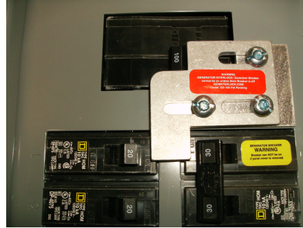
Homeline Generator on
