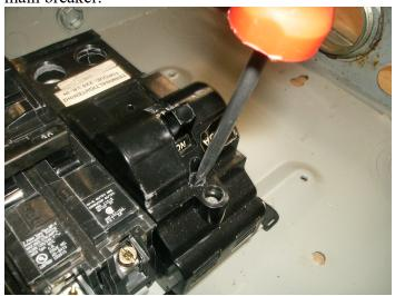
Step 3: Install new main breaker, install leads and retaining screw (see photo).
